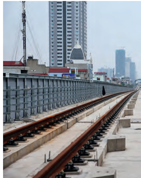
Energy-conservation measures were taken in the construction of the light rail, with uphill and downhill departure designs.
